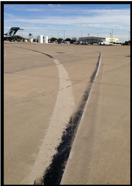
Grinding Left Waterblasting on Right
