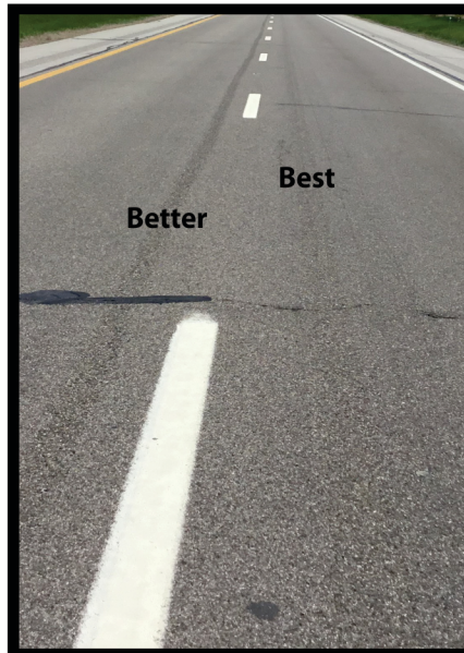
Water Blasting Better<>Best Highway Removal
